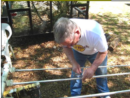
Above: When all else has failed, read the instructions... Below: Installing the linear loading wires
