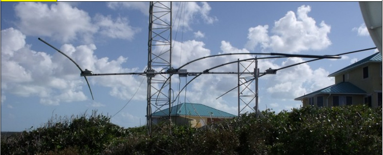
VP5DX SteppIR secured at 6 feet ABG until October
